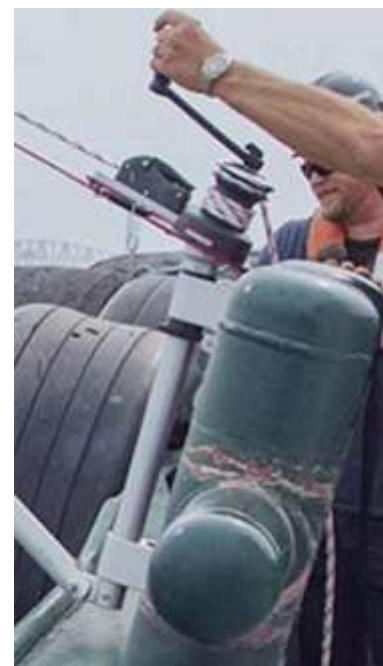
Image J6 The bitt dome top was welded on. Weld will be cleaned up where the davit will sit
